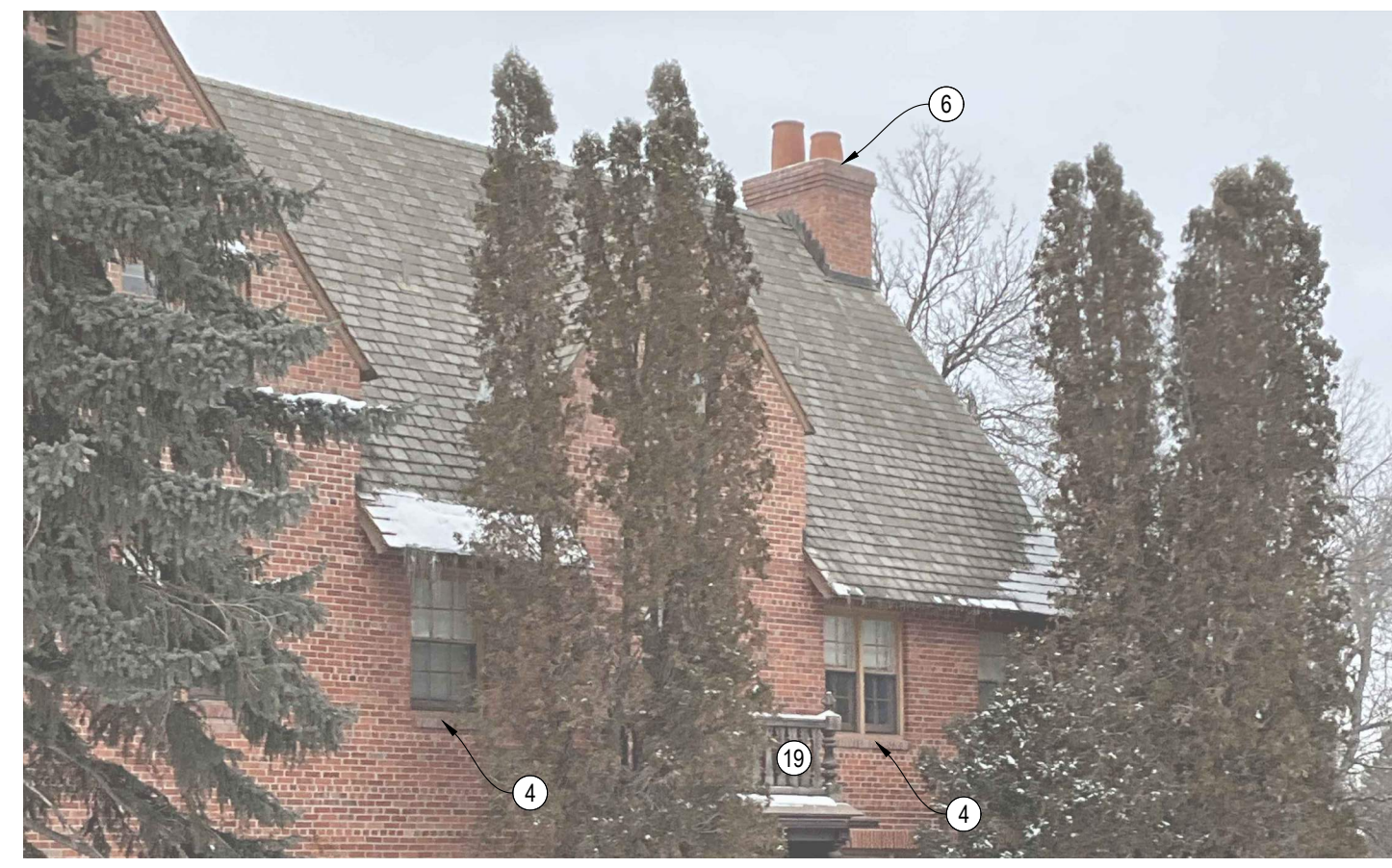
2 QUAD E EAST ROOF A2.3 : A4.6 PHOTOGRAPH
