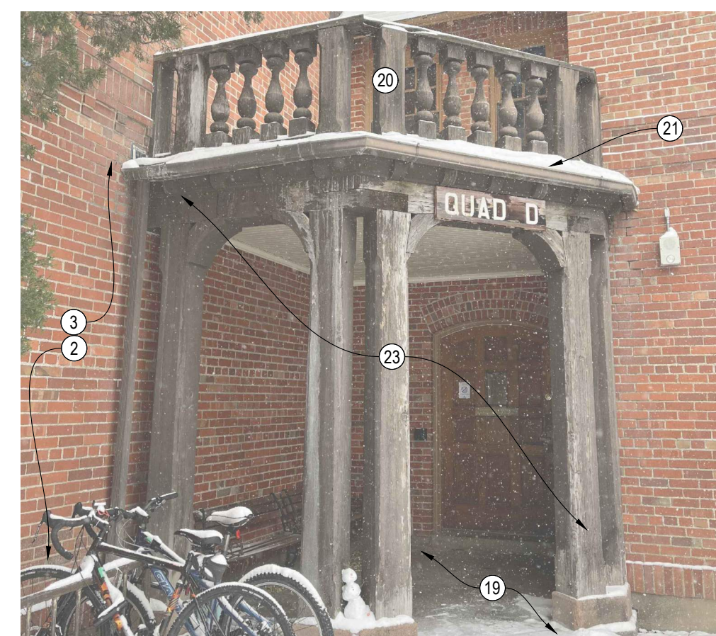
12 QUAD D SOUTH ENTRY A2.2 : A4.5 PHOTOGRAPH
