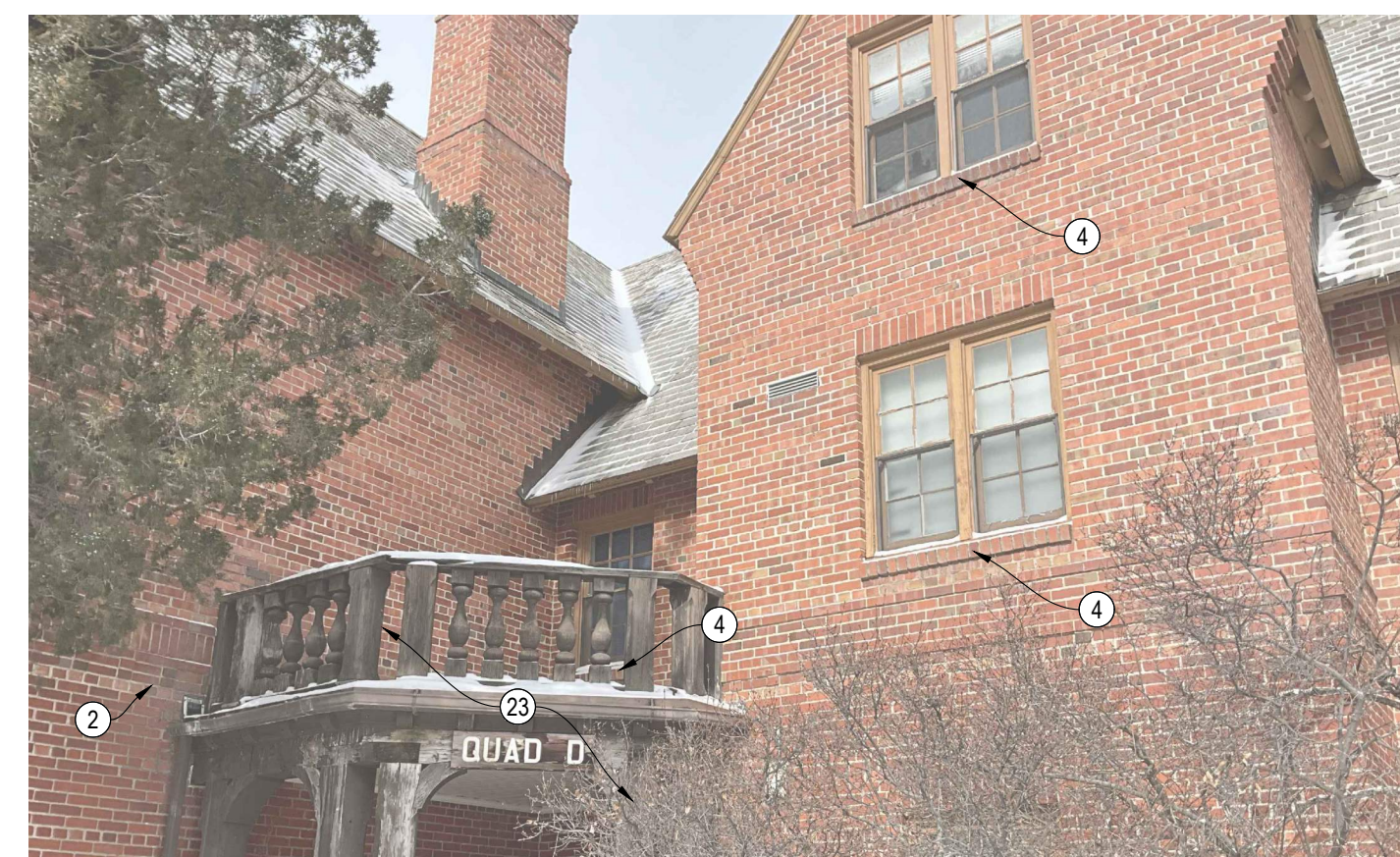
8 QUAD D SOUTH PORCH A2.2 : A4.5 PHOTOGRAPH
