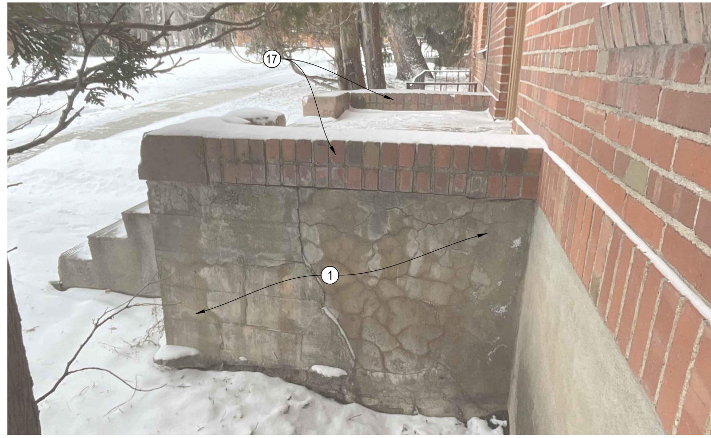
5 QUAD E CONCRETE STOOP A2.3 : A4.6 PHOTOGRAPH
