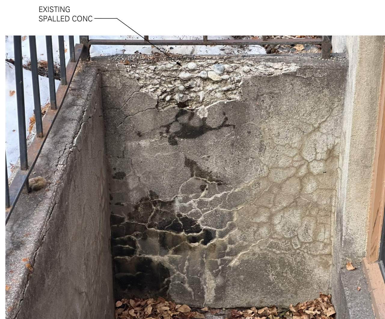
9 SPALLING CONCRETE REPAIR SCALE: 3/4" = 1'-0"
